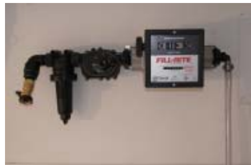
Water Meter Assembly
