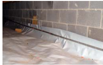
Conditioned Crawlspace
