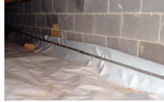
Conditioned Crawlspace
