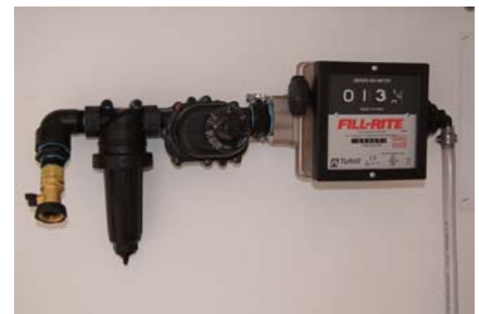
Water Meter Assembly
