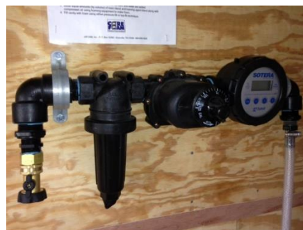
Water Meter Assembly
